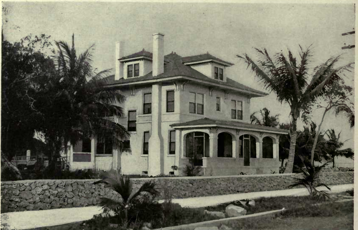
Residence of James MacRoberts, Miami, Florida. August Geiger, Architect, J. B. Orr, Stucco Contractor All stucco waterproofed with Truscon Waterproofing Paste, Concentrated.
